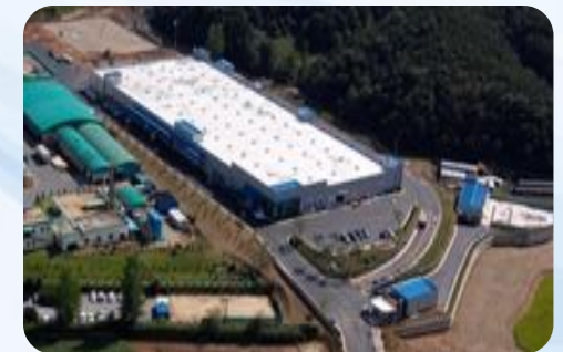
Coating & Rolling Facility: Yugu, South Korea
